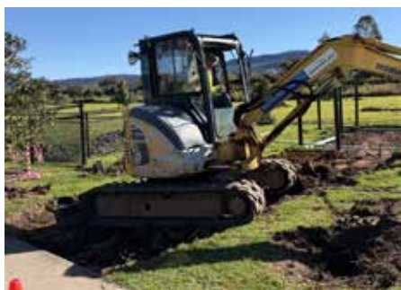
Club member Ken Hutt excavating the main gate entry which will be paved with engraved pavers sponsored by members of the community.
