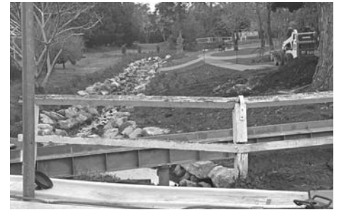
Alexandra Street Park footpath works
